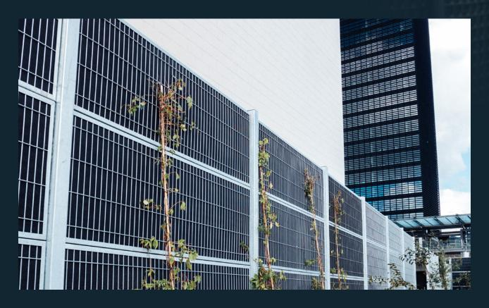
Noisecare fence has been developed as a special module. The fence consists of pre-assembled modules in standard dimensions with fixed heights and width per section, the design of the modules allows the noise fence to follow the natural bends and curves of the road. Any level difference in the terrain can also be offset so that the best noise reduction is achieved.
